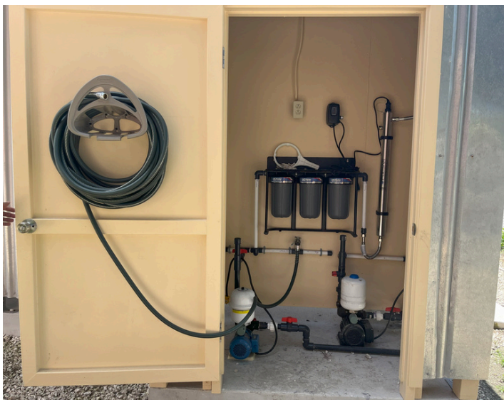
Compact water filtration system installed in a secure outdoor enclosure, featuring multiple filtration stages and a hose reel for convenient access.
